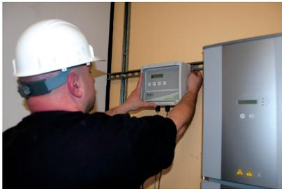
Mount the Management Unit (MMU) in a location that has access to an AC power source, a stable network connection, and proper cable connection to the Gateway. The MMU should be mounted between 3 and 5 feet above the ground. Mounting tabs are provided for installing on uni-strut or directly to a wall surface.
